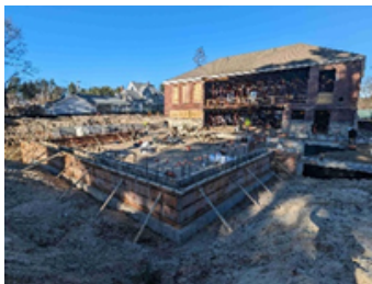
construction site with wood frame prepared for concrete pouring
