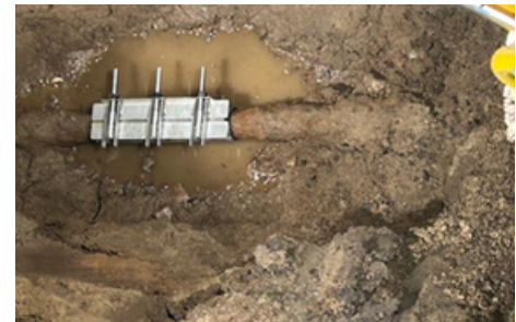
a hole in the ground with leaking steel pipe covered
