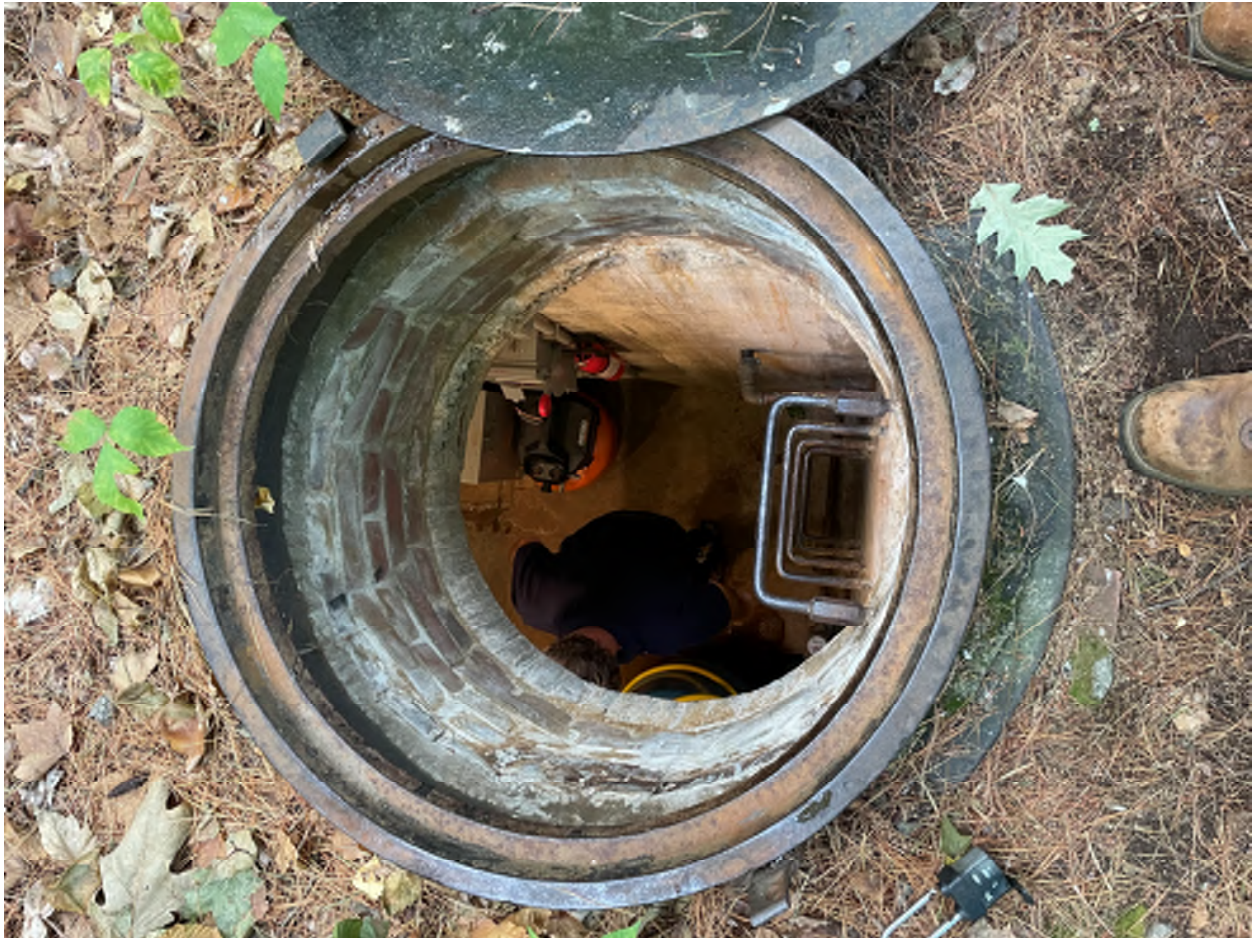
Photo 1 - Access manhole to underground vault
